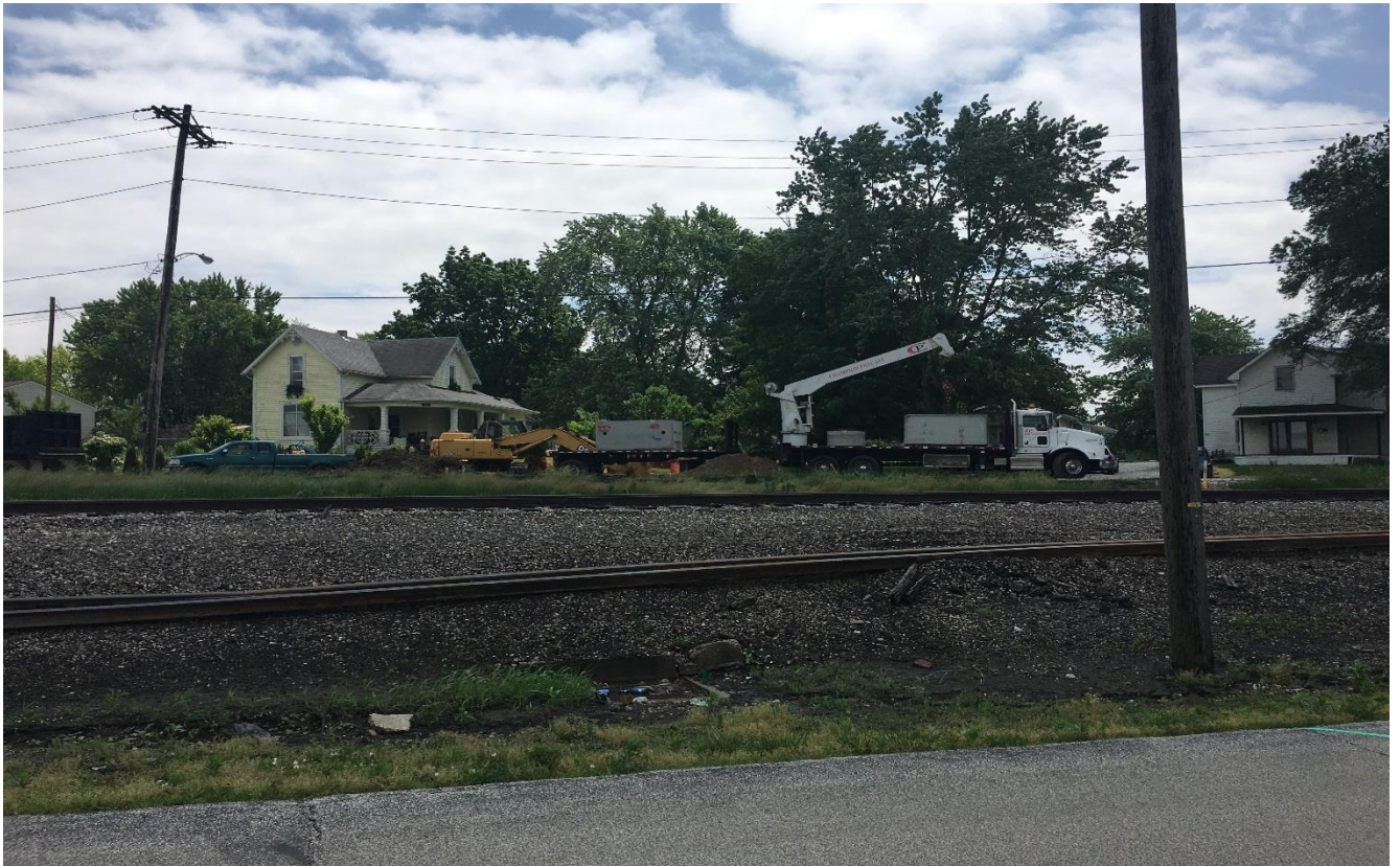
Delivery of ATT structure
